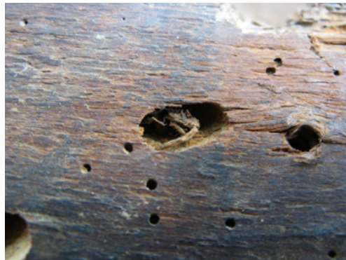
Figure 41. Remains of xylophagous insects in a support. Photographs: Cristina Salas.
