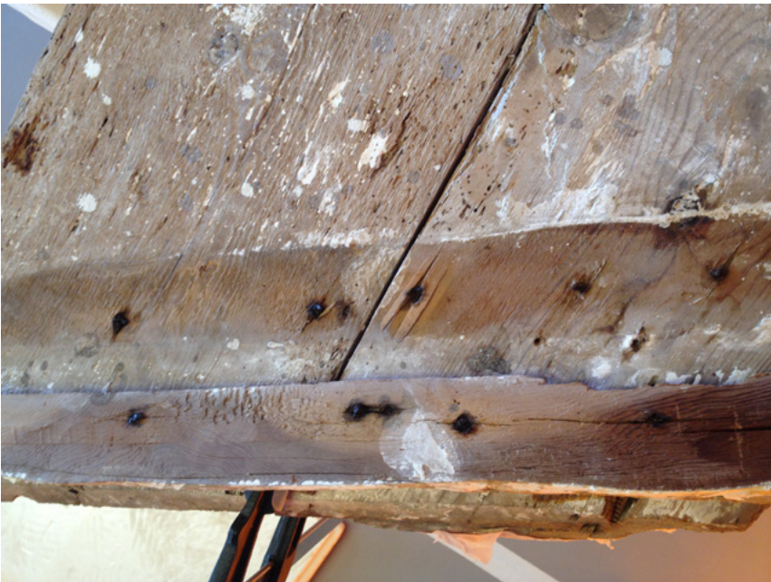
Figure 38. Effect of the oxidation of metal elements of a wooden support. Photographs: Cristina Salas.
