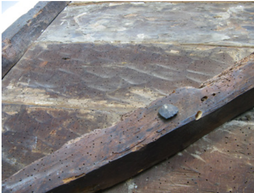
Figure 40. Effect of xylophagous insect infestation on a wooden support. Photographs: Cristina Salas.
