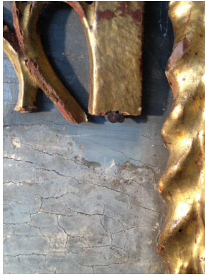
Figure 55. Example of the difference in condition of the pigments protected under the wooden moulding. Photograph: Cristina Salas.
