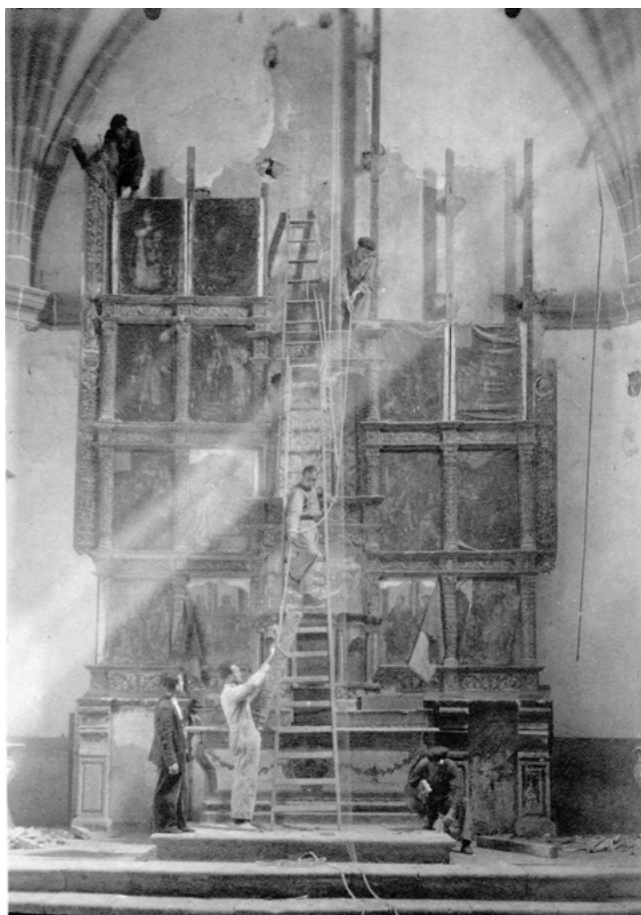
Figura 3. Disassembly of the altarpiece in the parish church of Balconete, (Guadalajara). Photograph: IPCE Photo Archive, Aurelio Pérez Rioja (1888-1949)
