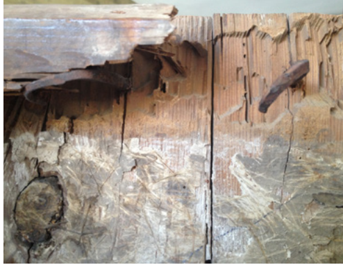
Figure 39. Beam damaged by pests, in which a wrought nail is exposed. Photographs: Cristina Salas.
