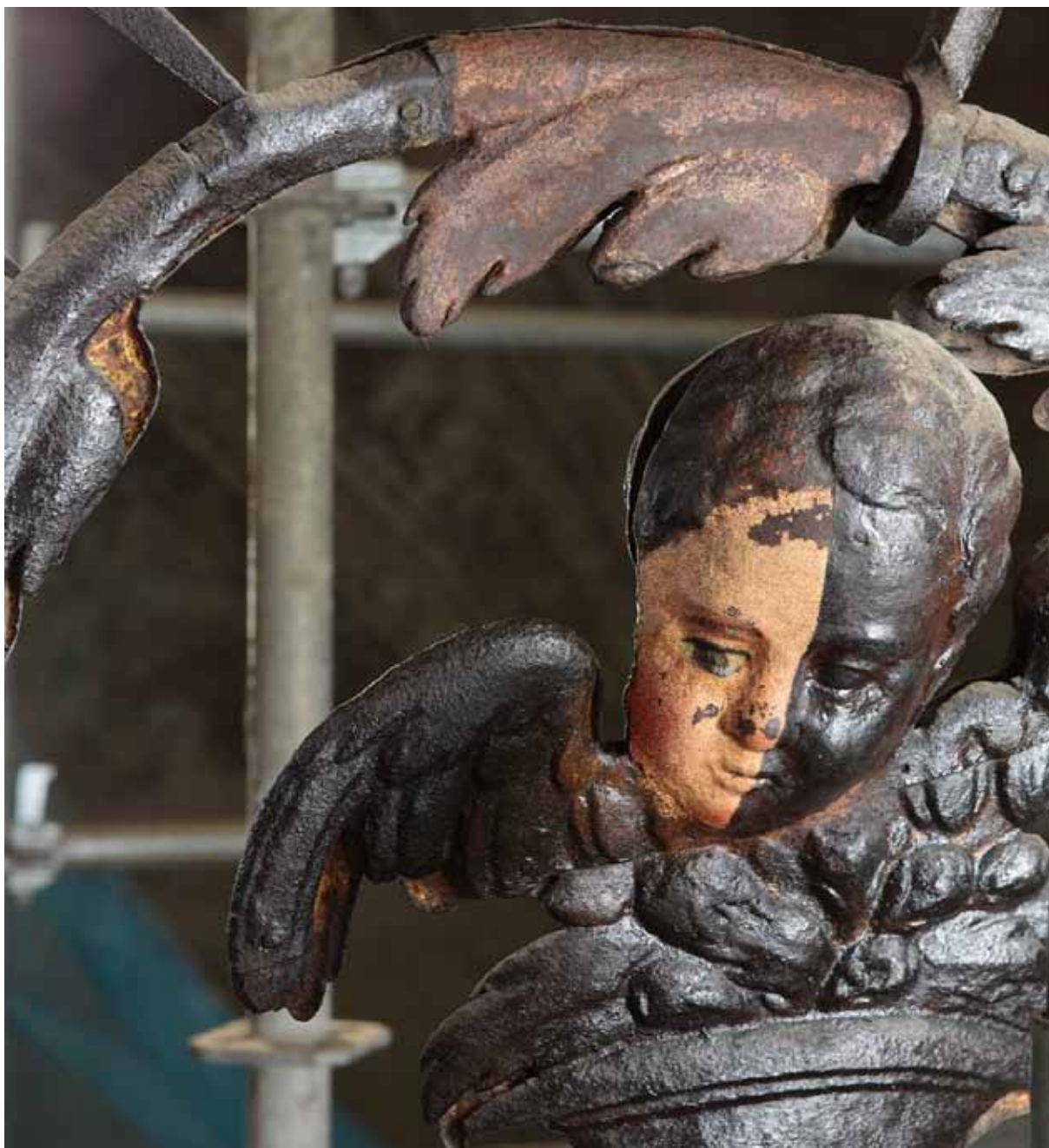
Figure 24. Chemical cleaning samples. Wrought-iron enclosure, the Scalas Chapel, Seville Cathedral.
